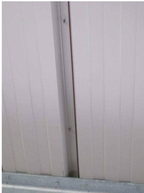
Foto 7.20: Zelftappende schroeven in de overlap van de dakplaten (TNO)
